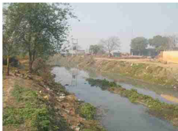
NTPC canal after removal of vegetation cover.
